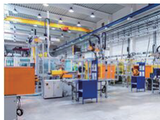
Embedded Production Equipment
